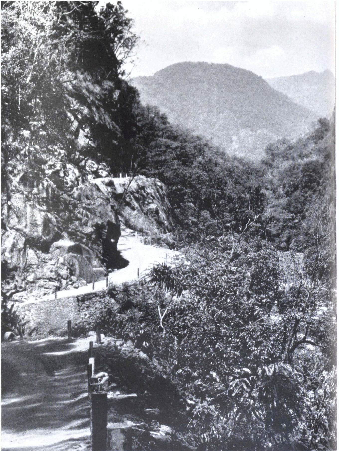
A scene on the new road, built by Army Engineers, connecting Ziro, headquarters of the Subansiri Frontier Division, the former 'Hidden Land', with the plains
